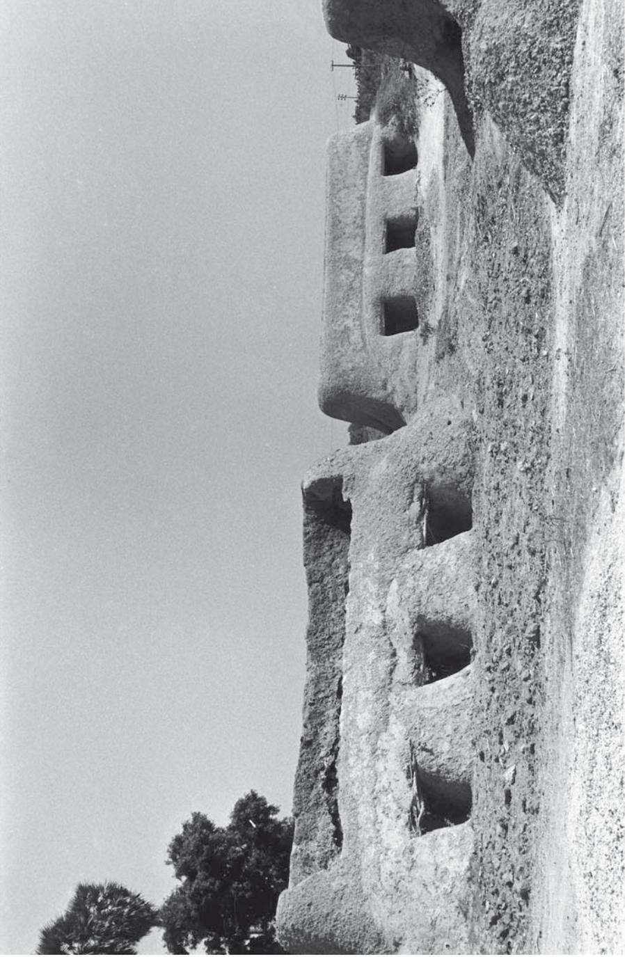
Ph. 47. Valdaaur, Tamil Nadu, lime ovens. The structure of the foreground is an empty oven. In the background is a cooling oven with the fire put out.
