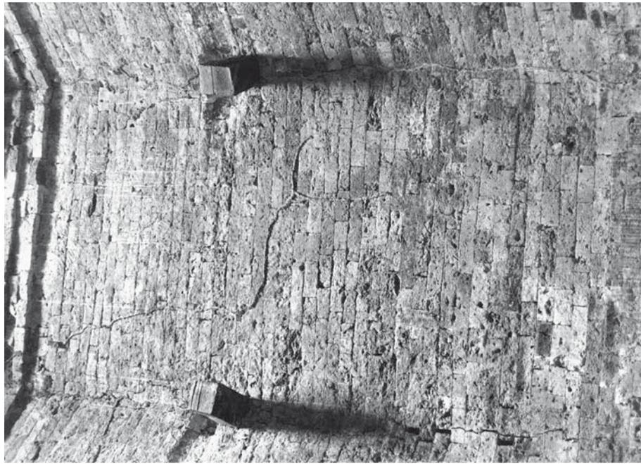
Ph. 35. Sambor Prei Kuk, inner wall of an octagonal tower made of brick, with sandstone hooks supporting the ceiling beams.
