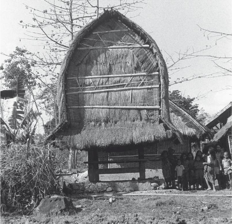
Ph. 21. Lombok, grain silo covered with roofing resting on screeds.
