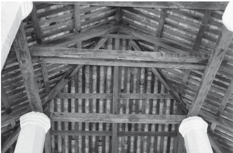
Ph. 19. Malaysia, near Lembah Bujang, mosque of Pangkalan Kakap, modern truss built over a radiating framework.
