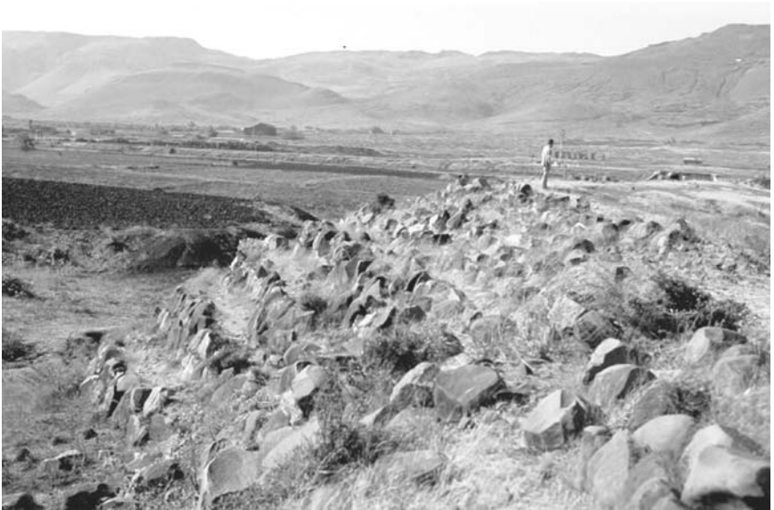
Figure 4.2 Masonry-Faced Embankment of an Abandoned Sixteenth-Century Reservoir in the Daroji Valley. The Sandur Hills, in the Distance, Show Scars from Recent Mining.
