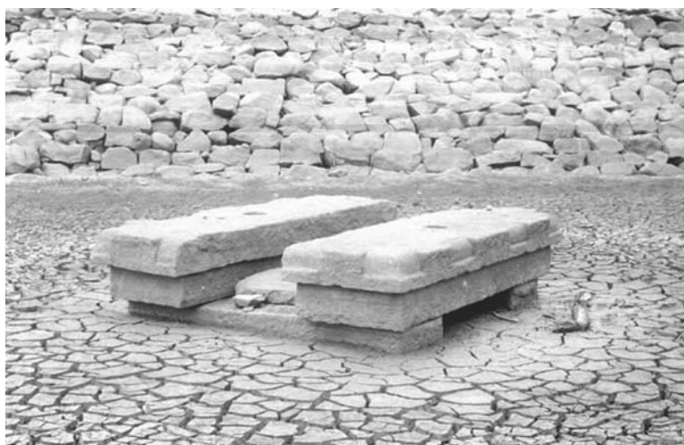
Figure 4.4 Avinamodugu Reservoir Sluice Gate Buried In ca. 3 Meters of Silt. Despite Extensive Renovations, This Sixteenth-Century Reservoir Now Operates at only a Fraction of its Original Capacity.
