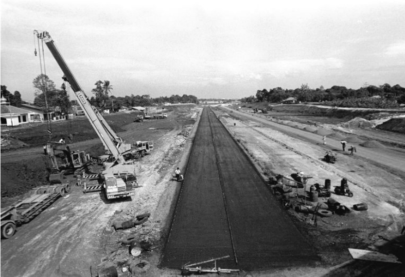
Figure 2.4 Construction of the Jakarta–Cikampek Tollway in 1986 ( Tempo /Anizar M. Jasmine).
