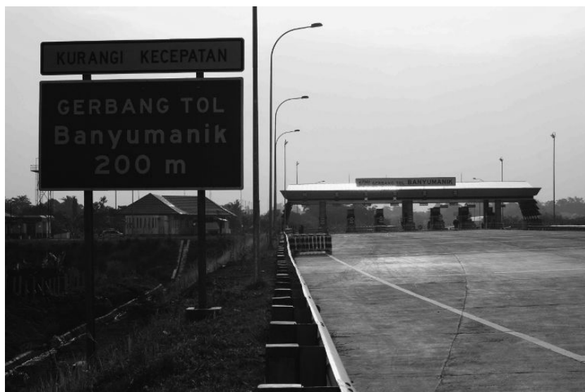
Figure 6.4 The Banyumanik Toll Plaza in 2011 where the Tirta Agung neighborhood once stood ( Tempo /Budi Purwanto).
