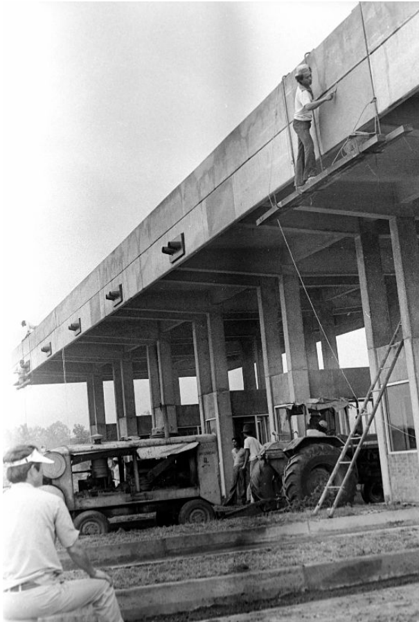
Figure 2.2 The building of the Jagorawi's toll plazas in 1971 ( Tempo / Eddy Herwanto).
